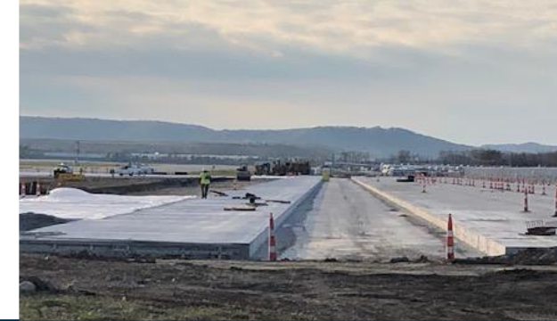
West Cargo Apron - Ramp 23 Construction $23.7 million
