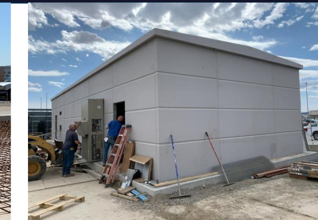
Terminal Electrical Switchgear Project $2.25 million
