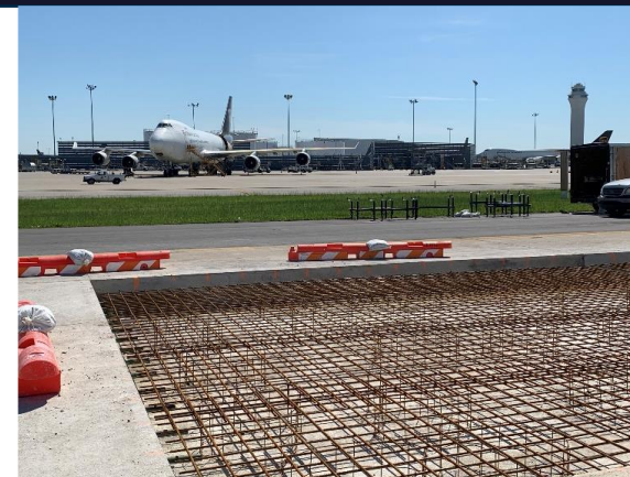
Runway and Taxiway Pavement Rehabilitation $23.5 million
